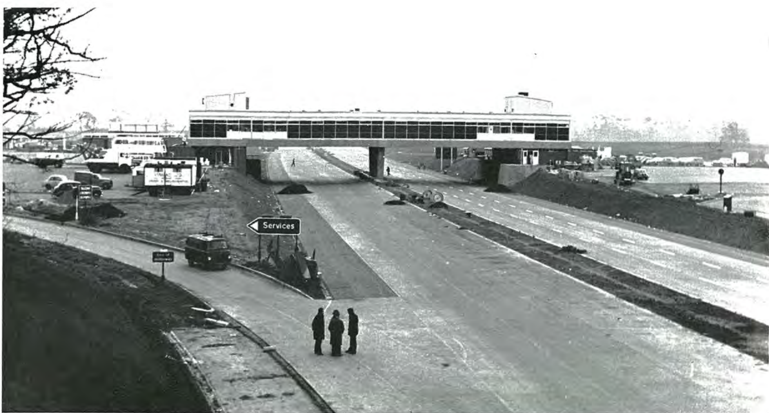
General view of the Service Area at Knutsford, when work was approaching completion.
