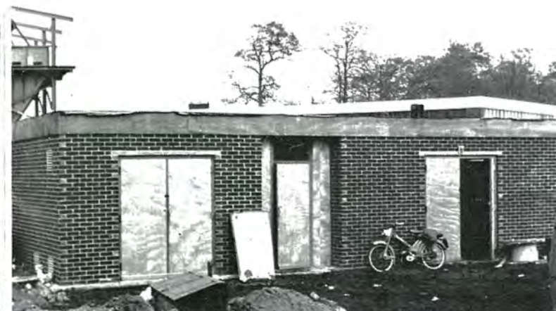
Below: The Service Area substation.
